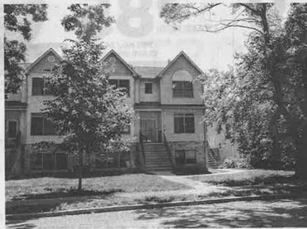
The building that houses the MLK Day Care program in Monsey. MLK Day Care was fined $2,500 in 2013 for violations including leaving children without competent care, leaving children in the care of other children, not having enough caretakers for infants and failing to cooperate with state inspectors. THE JOURNAL NEWS
